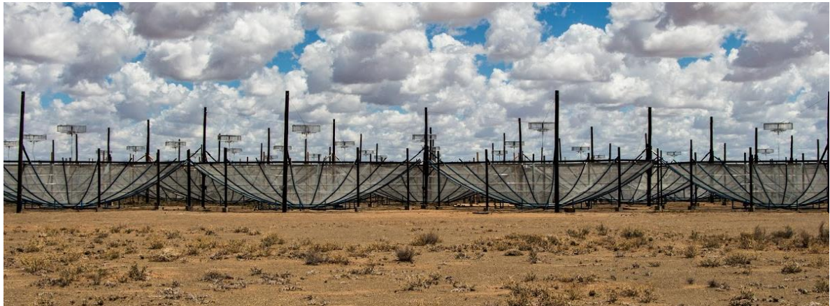
Figure 1: Part of the existing HERA installation
