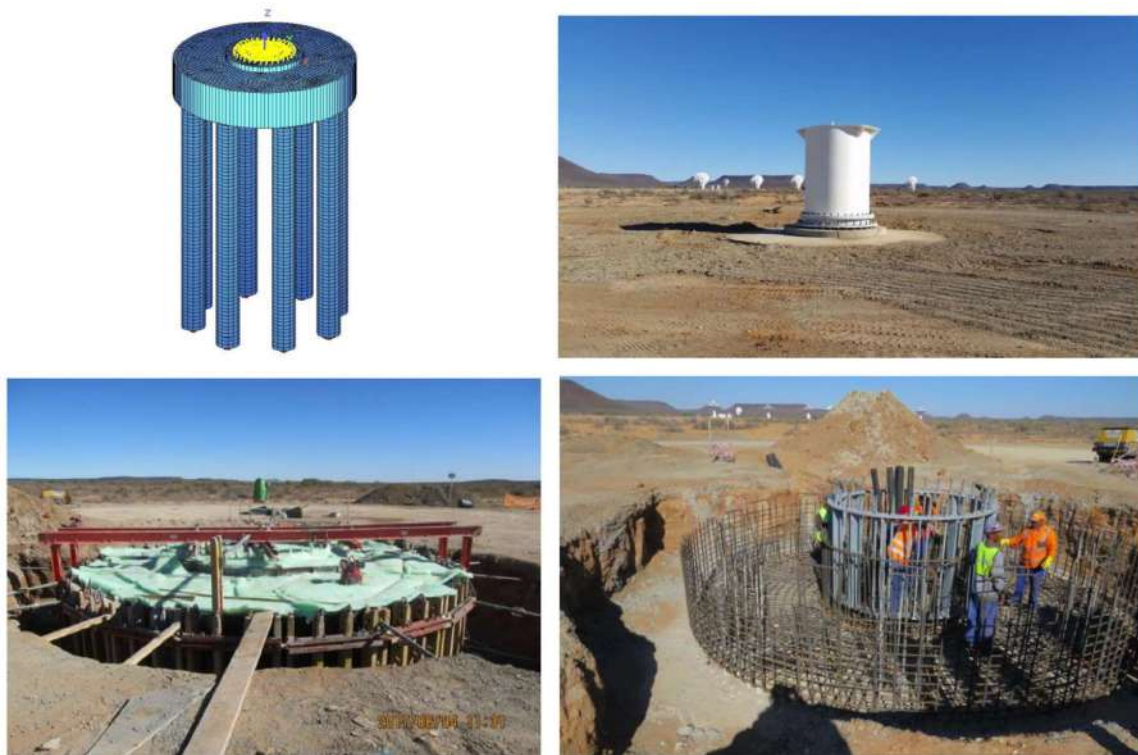
Figure 14: Model of Antenna Foundation (top left); Completed Foundation (top right); shutter work prior to concrete casting (bottom left); reinforcing steel for pile cap (bottom right) (Source: Gaea Enviro Pty Ltd, 2018).
