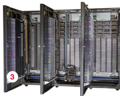
1. GNSS time transfer system
